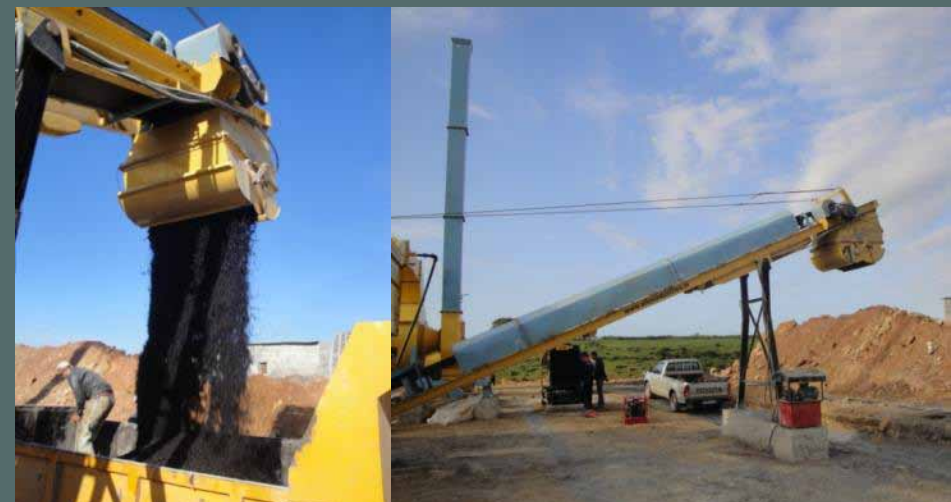
**FULLY COVERED LOAD OUT CONVEYOR TO REDUCE HEAT LOSS FROM HOT MIX
